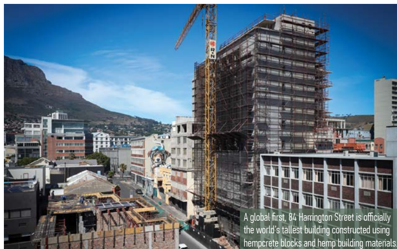
The lower density of the hemp blocks reduces the load of the walls on the foundations and therefore the cost of concrete.
