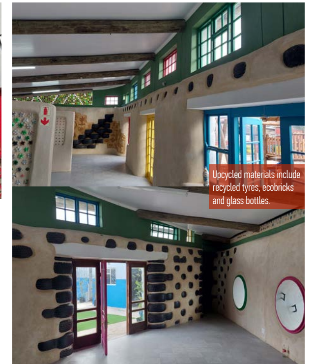
Ecobricks in walls inside classrooms.
