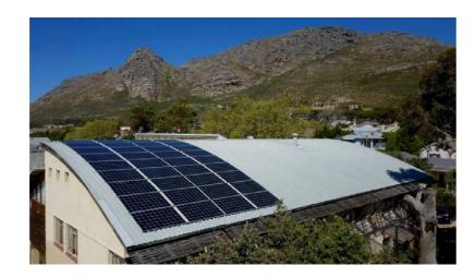
Designed and built back in 2004, the Green Building bolstered it's rooftop solar PV system in 2018, bringing it to net zero carbon status. The highly energy efficient building generates as much renewable energy as it consumes over a year.
