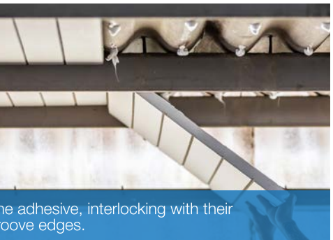
Appropriate adhesive is placed in blobs along the roof.
