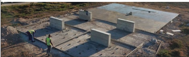
LPG Gas Farms Installations Plinths, Alternative Energy: Coega-PE/ Easigas/MM Engineering
