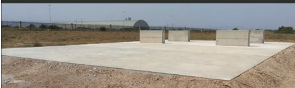
Light-Weight Polystyrene Slabs, Energy Efficient Using 60% Less Concrete: Dainfren Valley Estate
