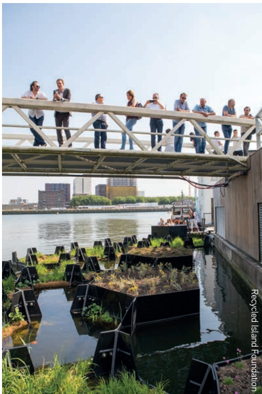
LEFT: The Recycled Park in Rotterdam, Netherlands, is constructed from floating islands moulded from plastic litter retrieved from the New Meuse River. The islands are filled with soil and plants, thus attracting local biodiversity, and creating a shelter for fish at their bases. RIGHT: Bosco Verticale (Vertical Forest) by Stefano Boeri Architetti in Milan, Italy, is a pair of residential towers that incorporate actual trees and shrubs in the architectural design – attracting local urban biodiversity.
